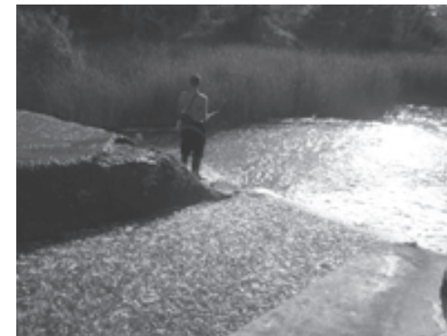
ramp and pool
